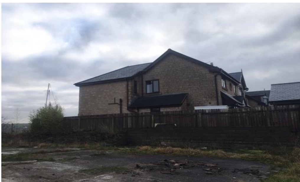
Case officer site photograph, taken 23 rd October 2020 – Gable of No.10 Tower Court, first floor windows on front and gable.
